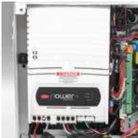
Built-in variable frequency drive.
