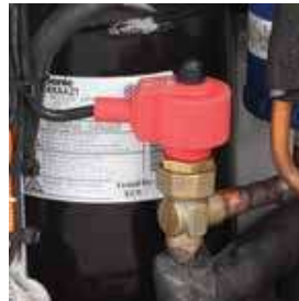
Electronic expansion valve for precise control of superheat.
